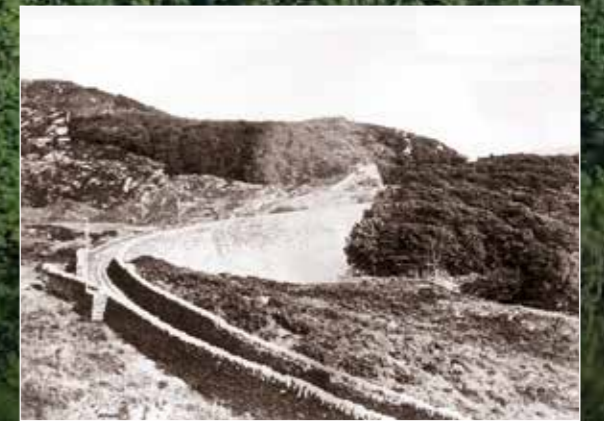
Strengthened with stone buttresses in 1887 and 1890 at the cost of £1000, the wall has, over the past 130 years, transported thousands of tonnes of slate as well as thousands of passengers safely across the ravine.
